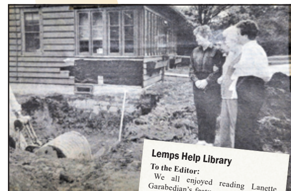
The expansion project was finally approved and the ground is being broken for the new addition in May 1989.
